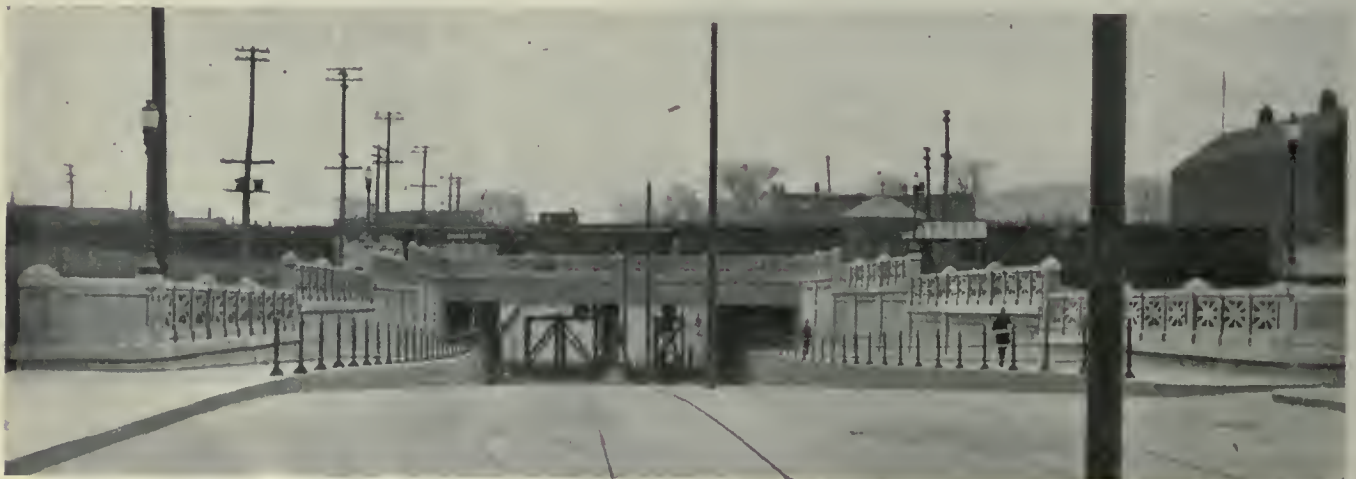
North end view, Park Avenue Subway, Montreal, P.Q.
